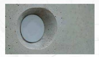
The water swellable sealing products by Vexcolt are based on the unique Active Sealing Technology. Our products expand on contact with water. This is how they create an active seal to combat moisture infiltration. The Vexcolt products are self-correcting and thus also sealing the unevenness and imperfections of the concrete.
